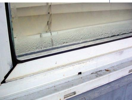
Condensation forms first on the coldest surfaces of a room, usually on glass surfaces of windows and doors.
