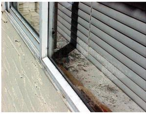
Evidence of problems resulting from condensation can be seen on the interior window sill.
