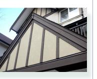
Fibre cement board is a composite material comprised of wood fibre, sand, and cement. The product is painted, and is available as a panel, siding or shingles. Maintenance and renewal activities are focused on cleaning and repainting.
