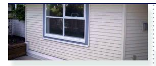
Vinyl siding is made from plastic (mostly polyvinyl chloride) and is intended to simulate the appearance of wood siding. A variety of colours and textures are available. Maintenance is focused on cleaning.
