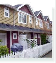
Wood siding, typically cedar, is lapped to keep water on the outside of the wall. Maintenance and renewal activities are focused on cleaning and refinishing, typically with paint or stain.
